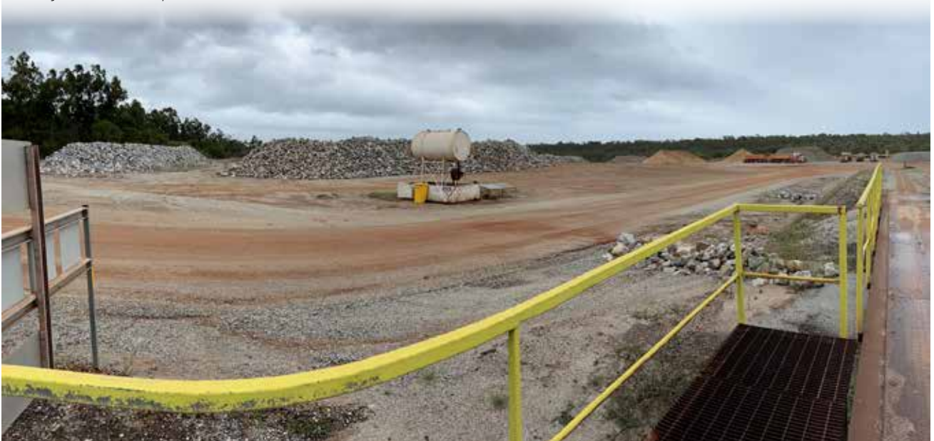
Quarry rock stock piles
